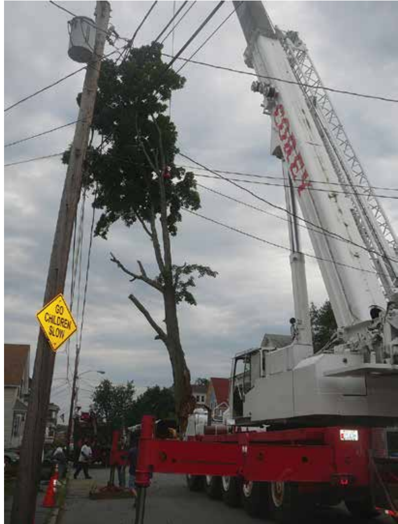
Phase-to-phase faults can be caused when any object connects two phase wires.
