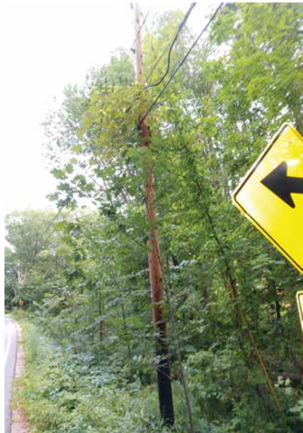
Vines growing up utility poles or trees can create an electrical hazard.
